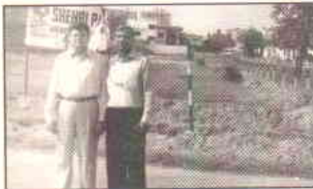
Work in progress: Barbed wire/bamboo fencing erected
